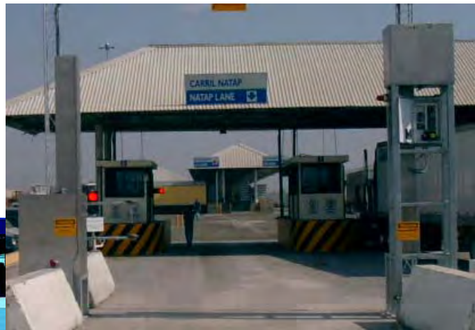
Figure 7-5 Portal VACIS - Gamma Ray Imaging System
